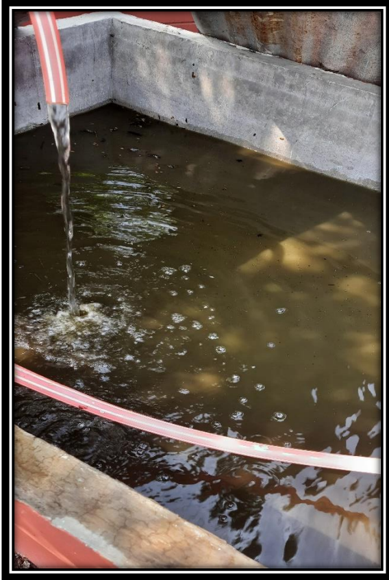
Photos of Slurry Tank
